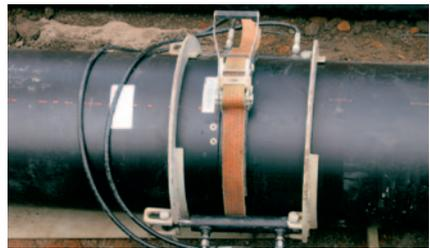
5. Attachment of tensioning tool (in this case a strap) to reduce the joint width and exert required pressure for joining.
