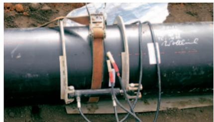
6. Connection of 40 V standard automatic welding machine for electrofusion sockets to existing 4 mm contacts.
