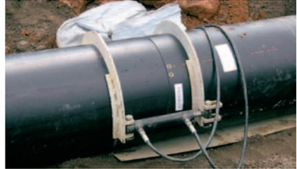
4. The two pipe ends are brought together by means of hydraulic force.
