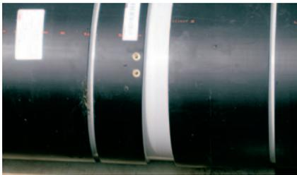
2. Insertion of spigot end into socket on a carefully prepared, clean surface.
