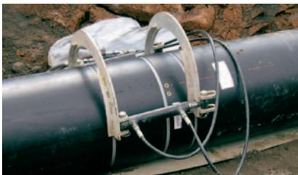
3. Adjustment of hydraulic clamping device. Clamping collars fit into the appropriate grooves.
